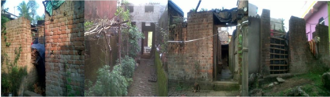
Photo2. Tikarpada Sahi partly constructed DU's
