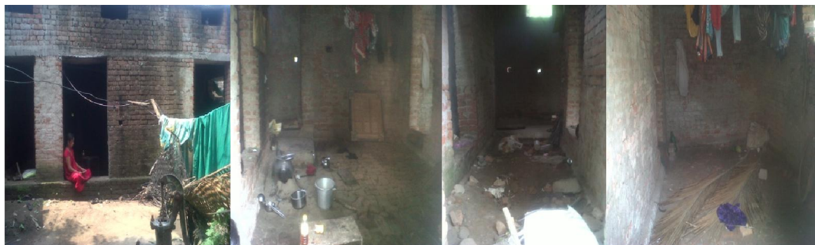
Photo 6. Partly Constructed DU's in MangalaSahi NS Depot
