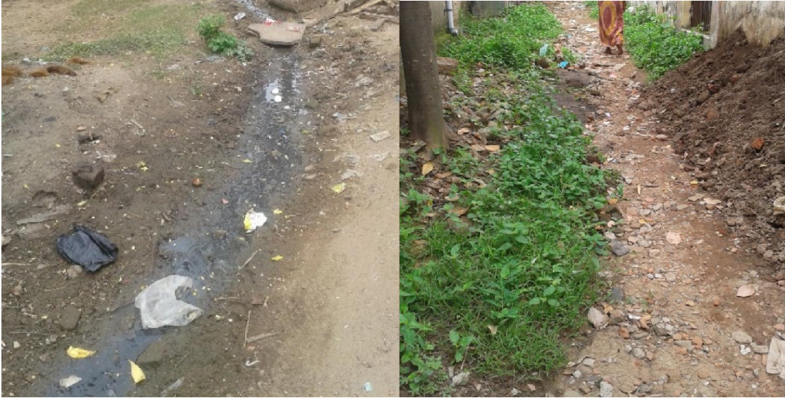
Photo 16. Dirt track instead of paved path in Tikarpada slum
