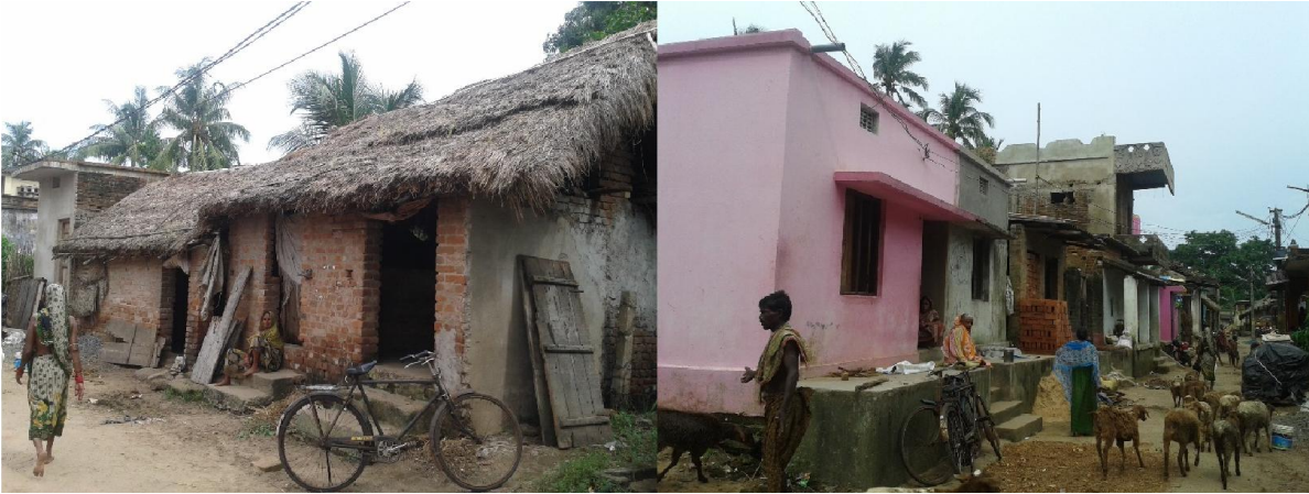
Photo 17 . Matitota Phase 1: Houses constructed with money borrowed from local sources
