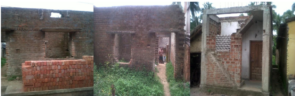
Photo1. Partly constructed DU's
