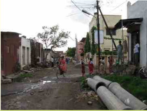
Pipes to be laid for underground drainage in haddawadh areas
