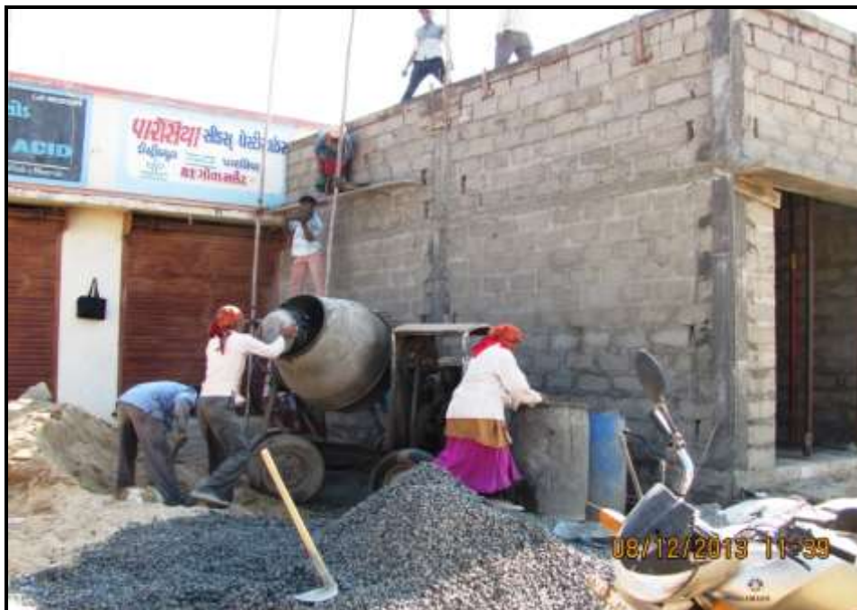
Figure 3.3-7 Construction labourers at a site near Geeta Market, Bhuj
